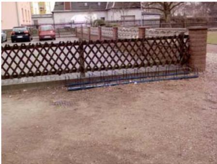
**Foto: This trellis-work fence in front is inappropriate, because it encourages to climb, it has laces and there are head-trapping hazards (a childs head can be trapped in a square between the pickets). The wall in the background with concrete elements is also easy to climb on and it has head-trapping hazards.**
